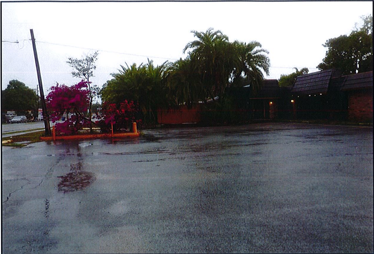
Photograph No. 1 View to the west along the southern Subject Property boundary. Note 46 th Avenue North to the left.
