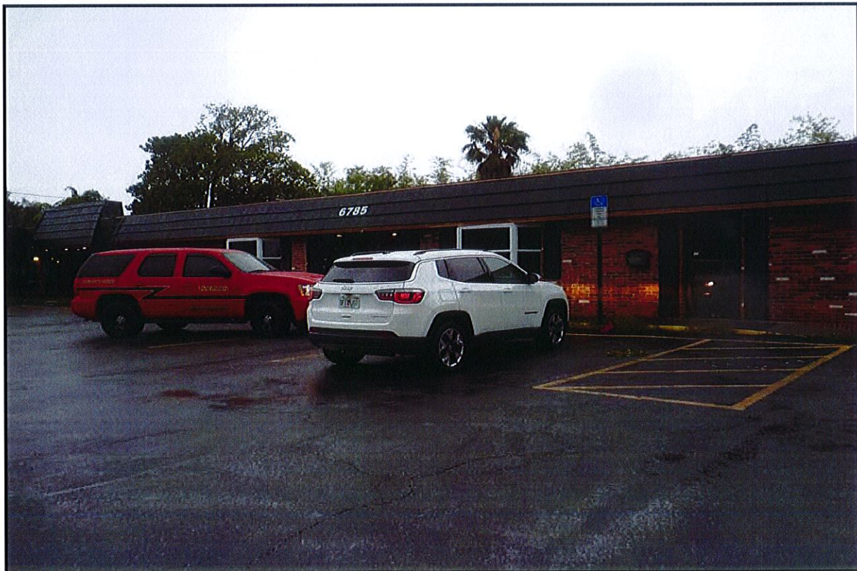
Photograph No. 2 View to the northwest of the front of the onsite multi-tenant office building and paved parking area.
